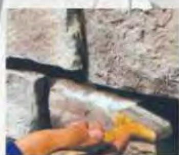
6: THE JOINTS ARE BRUSHED.
