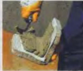
2: APPLY MORTAR TO THE BACK SIDE OF STONES ALSO.
