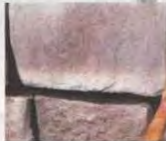
5: THE JOINTS ARE POINTED.
