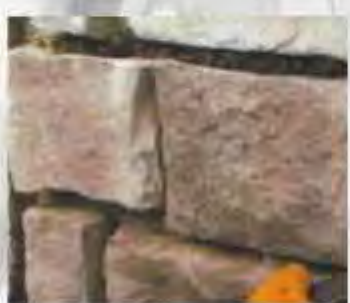
4: THE JOINTS ARE GROUTED.
