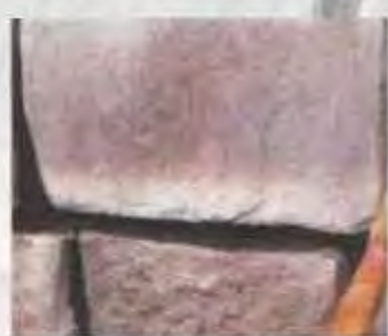
5: THE JOINTS ARE POINTED.
