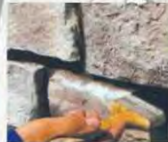
6: THE JOINTS ARE BRUSHED.
