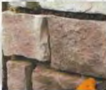
4: THE JOINTS ARE GROUTED.
