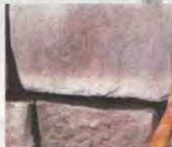
5: THE JOINTS ARE POINTED.
