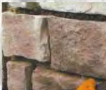
4: THE JOINTS ARE GROUTED.
