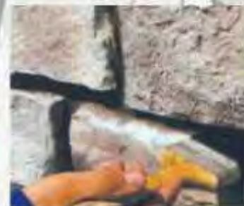
6: THE JOINTS ARE BRUSHED.
